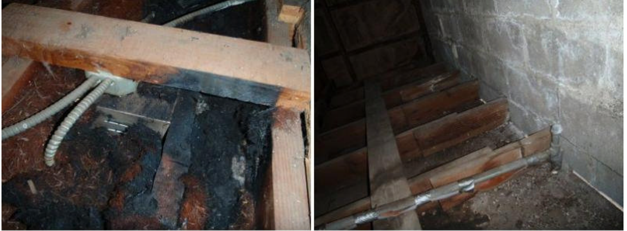
Rafter framing with solid wood sheathing.
