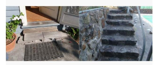
**Steps into the house are higher than standard.** In some cases, loose blocks have been set in front of the doors, but these are likely to move and are potentially hazardous. I recommend installation of proper steps at all exterior doors. Ideally, all steps would have easily gripped handrails.
