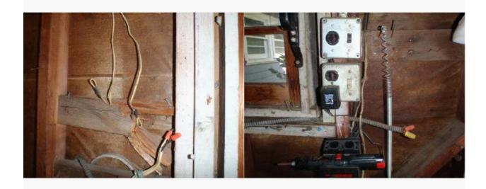
**Electrical wiring is unsafe and nonstandard.** Terminated wiring and open junction boxes are present. Corrections should be made by a licensed electrical contractor concurrently with other repairs noted in this report.
