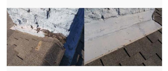
**Asphalt patching compound (mastic) has been applied to the chimney flashing.** In addition, this flashing is older and nail holes are present. Decayed wood and evidence of leaking was found in the attic adjacent to the chimney. This flashing is likely to leak and I recommend replacement by a licensed roofing contractor.
