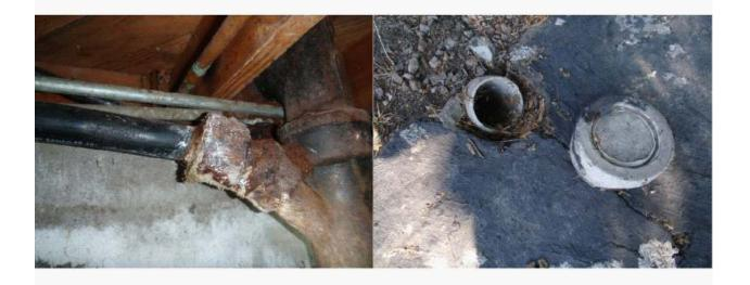
Where visible, waste lines are ABS (plastic) and galvanized steel.
