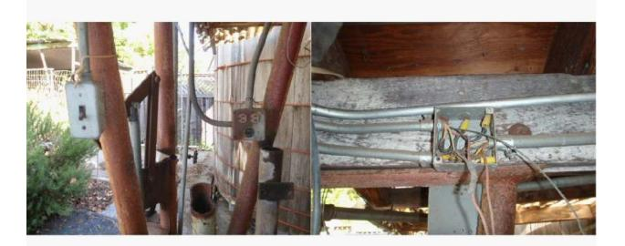
**Electrical wiring is unsafe and nonstandard.** No cover plates present on some junction boxes, nonmetallic sheathed cable has been used, loose wiring is not secured/hanging down and receptacle outlets are not GFCI protected. In addition, receptacle outlets do not have waterproof exterior covers. A licensed electrical contractor should be hired to make any needed repairs or corrections.
