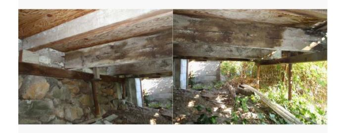
**The shed structure is not well supported/constructed.** The metal support posts are leaning. I recommend removal or resupport of this structure.
