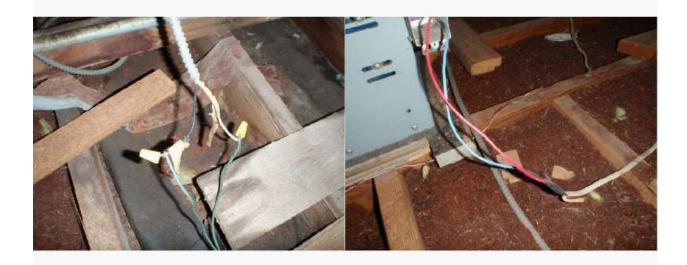
Improper and unsafe wiring was found at areas throughout the attic. Terminated electrical cable with exposed leads, unprotected electrical splices, open junction boxes and individual conductors were observed at areas throughout the attic space. A licensed electrical contractor should be hired to make any needed repairs or corrections.
