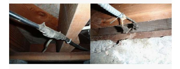
**Improper wiring was found in the crawlspace area.** Porcelain light fixtures are not secured to junction boxes and electrical splices are not enclosed in junction boxes. Corrections should be made by a licensed electrical contractor concurrently with other repairs noted in this report.
