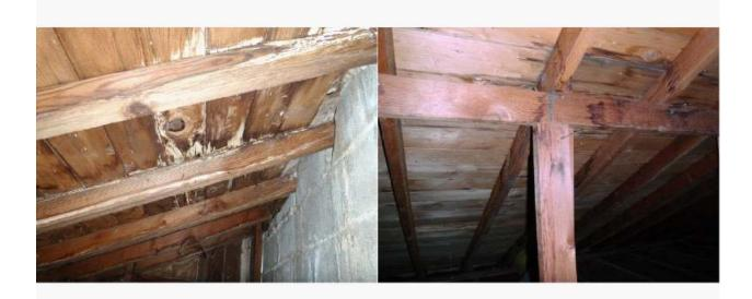
Moisture staining was found on the roof sheathing at various areas throughout the attic. While it is likely that most of the leaking has been corrected with installation of the current roof covering, the area adjacent to the chimney has some damage and may have more current leaks. Please refer to the roof/flashing section of this report for related information.
