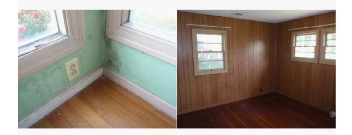
**Evidence of leaking was observed adjacent to the living room and south bedroom windows.** This is likely due to active leaking. The exterior of this window should be reflashed or resealed, as needed. Unable to determine the condition of enclosed framing without destructive testing. This should be reviewed by a licensed pest inspector for any wood damage.
