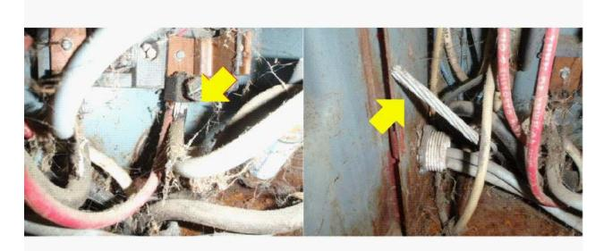
**Multiple wires are connected to a single circuit breaker terminal connection where only one wire should be connected.** This can prevent the wires from having positive contact with the connector which could lead to arcing or shorting. This is normally corrected by installing additional circuit breakers. Any corrections should be made by a licensed electrical contractor.
