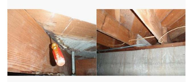
2x8 wood joists with solid wood sheathing.
