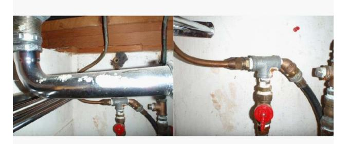
**Plumbing under the sink is deteriorated.** No leaking noted at time of inspection. Please refer to the plumbing section of this report for related information.
