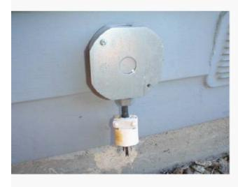
Switches and wiring have been pulled-out of electrical boxes adjacent to the tall carport and the pool steps. I suspect other unsafe and nonstandard wiring is present as well. A licensed electrical contractor should make repairs or corrections concurrently with other electrical repairs.
