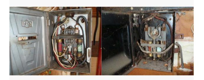
Other, older fuse panels are present in the garage. I recommend removal of these panels and properly removing/terminating the wiring/conductors.
