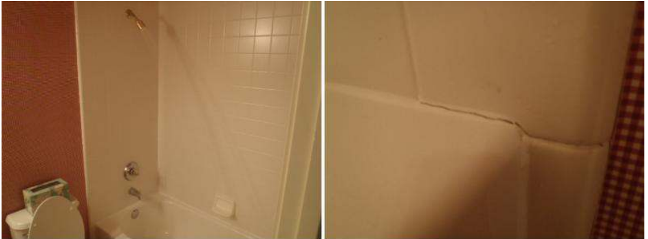
Tile surround walls with a fiberglass tub.
